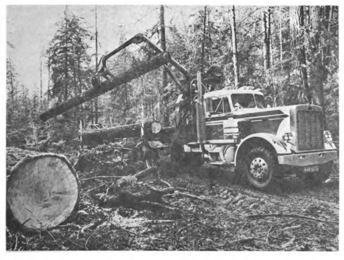
Figure 7-29. Truck-mounted grapple.
